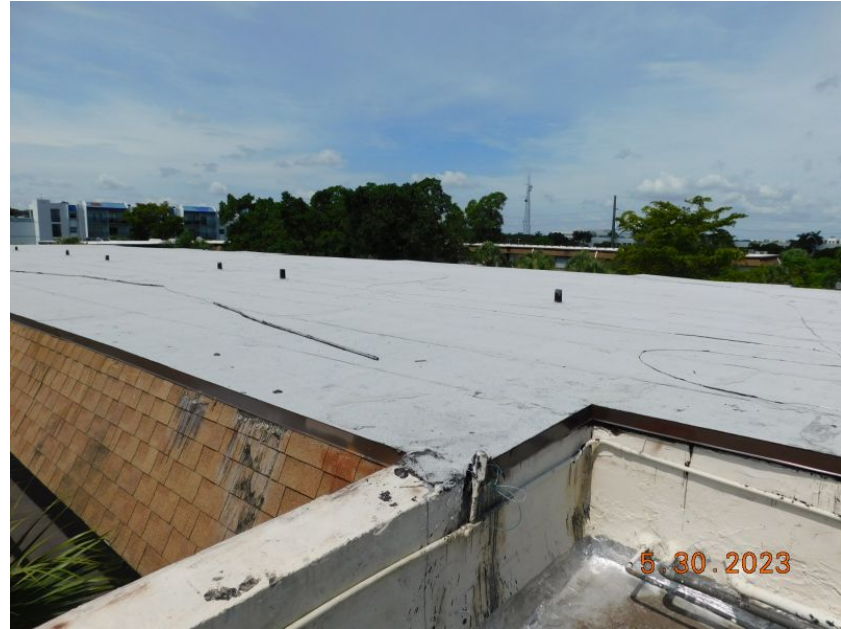
Built Up/Rolled Asphalt (Flat) Roof Covering
