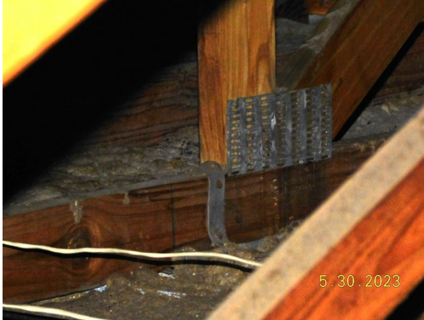
Metal Connector with 1 Nail on the Front Side & 2 Nails on the Opposing Side
