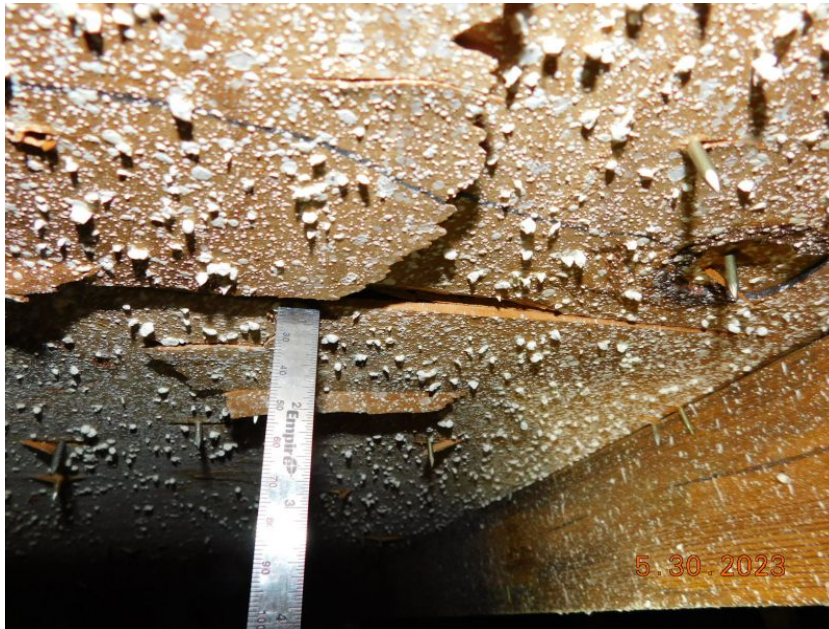
19/32" Deck Thickness Confirmed
