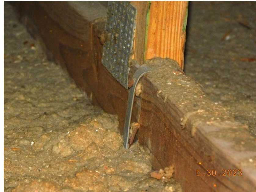
Metal Connector with 1 Nail on the Front Side & 2 Nails on the Opposing Side
