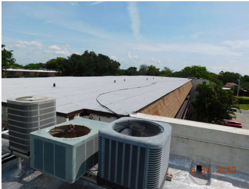
Built Up/Rolled Asphalt (Flat) Roof Covering
