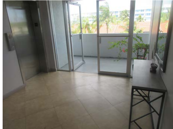
ELEVATOR LOBBY, DECK
