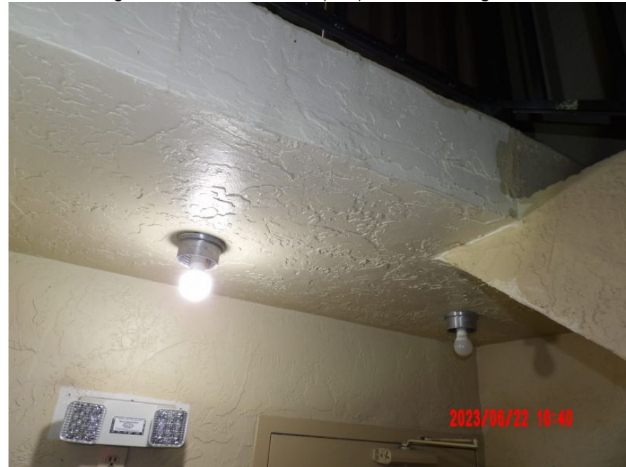
Reinforced Concrete Roof Deck
