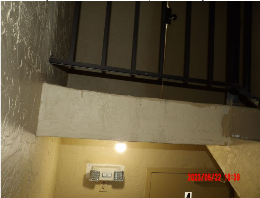
Reinforced Concrete Roof Deck
